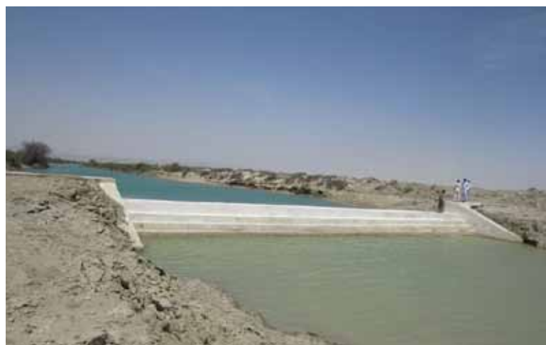
Diversion wall constructed under GLLSP Project, Gwadar
