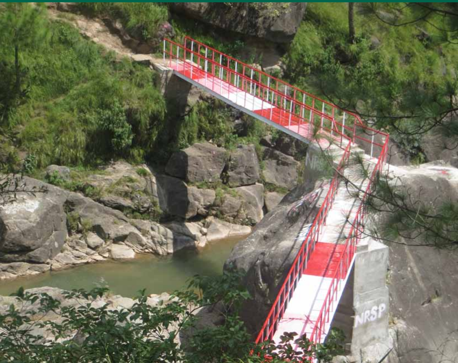
Foot Bridge constructed under EU-funded Project in District Kotli, AJK
